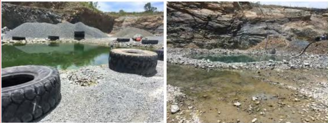
Figure 4-2 Quarry Pit sump waterbodies and pumping infrastructure
