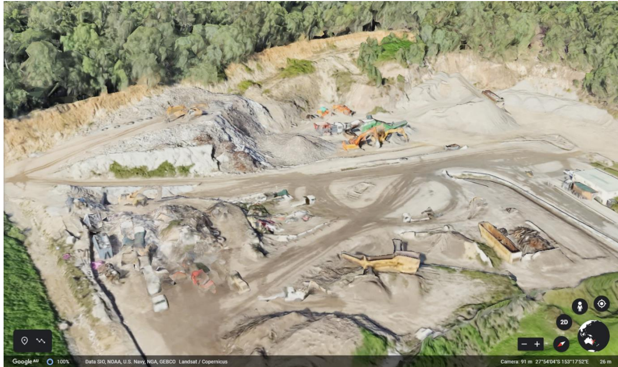
Attachment D4 - JJ Richards quarry and recycling operation (241 Tamborine Oxenford Road)
